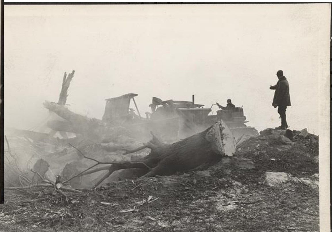
Bulldozer Pushing Tree into Fire ~ Clearing Reservoir Site ~ Cont. 61 ~ 1-26-39 ~ Photo Pike ~ (6) 1
