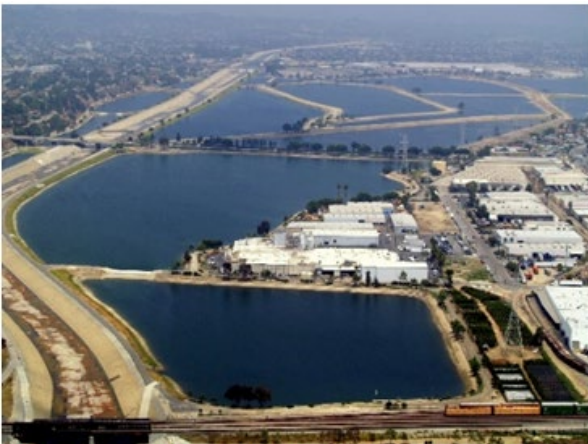
Aerial photos of the LA County Department of Public Works Rio Hondo Spreading Grounds
