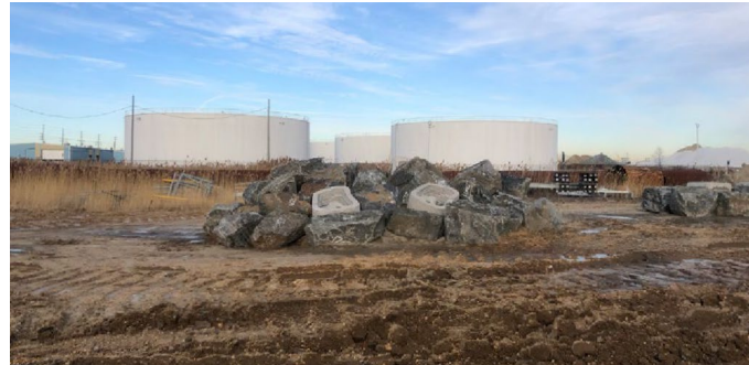
NORTH AMERICAN AGGREGATES Perth Amboy, NJ
