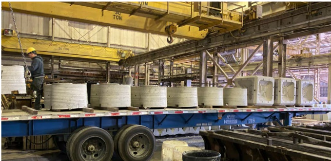
NJ PRECAST PLANT Ewing Township, NJ
