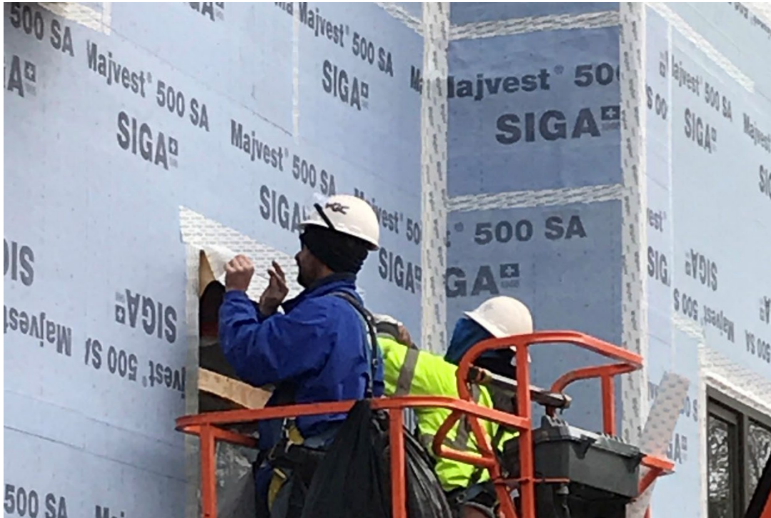
Air Barrier Taping from Exterior
