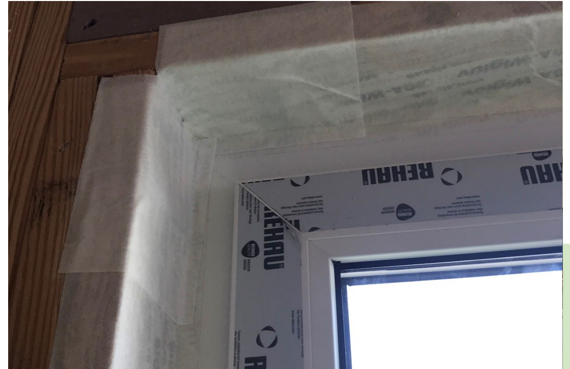
Window Flashing from Interior
