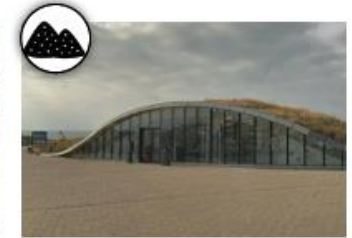
Parking Structure Built into Dune System
