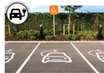
Electric Charging Stations
