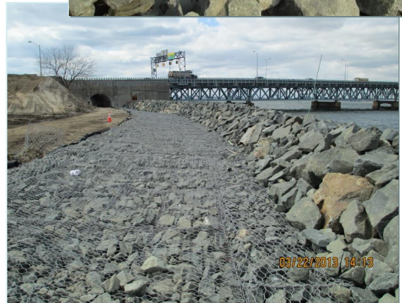
Restored abutment at Cross Bay Bridge
