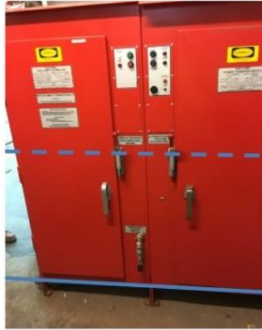
Figure 16: Building Systems – Fire Pump Control Unit
