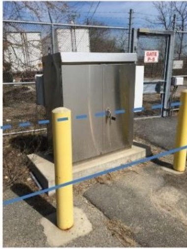
Figure 19: Blue Line Operations Yard Catenary Controller and Disconnect Switch
