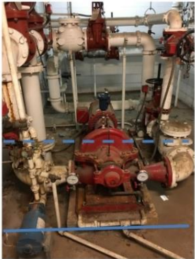
Figure 17: Building Systems – Barn Fire Pump
