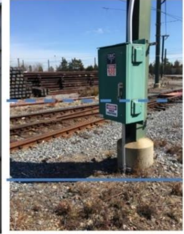
Figure 19: Blue Line Operations Yard Catenary Controller and Disconnect Switch
